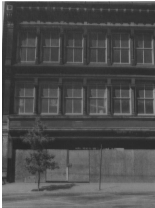
Figure 9. The MacRae Building-Otterbourg's Iron Front Men's Wear Depot, located at 25 North Front Street in downtown Wilmington, North Carolina. The structure is a Renaissance Classical iron front building and is an unusual find in North Carolina. ("MacRae Building," Wilmington, North Carolina: An Architectural and Historical Portrait , Tony P. Wrenn, with photographs by, Wm. Edmund Barrett).
